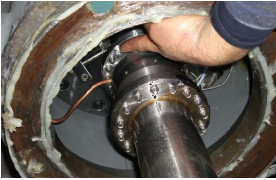
Figure 17. Weight installed on shop test coupling
