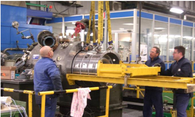
Figure 27. HP bundle removal after MRT
