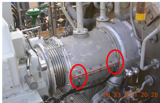
Figure 48. Torsional measurement system
